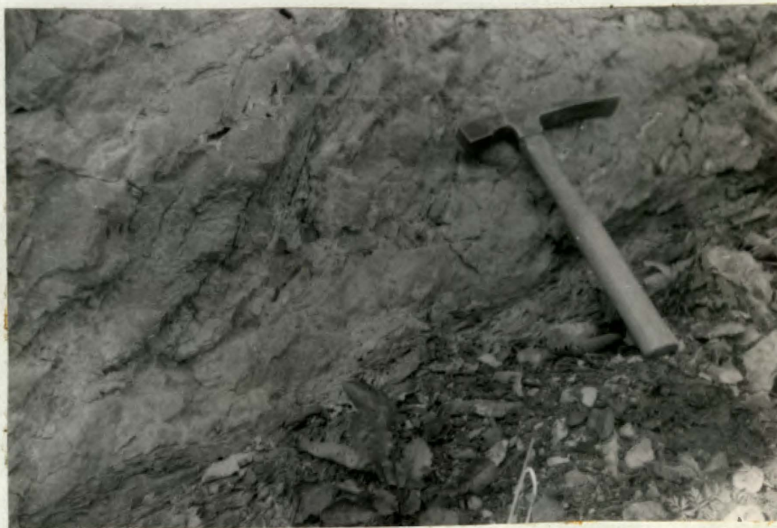
Figure 14. Closer view of fault shown in Figure 13.
